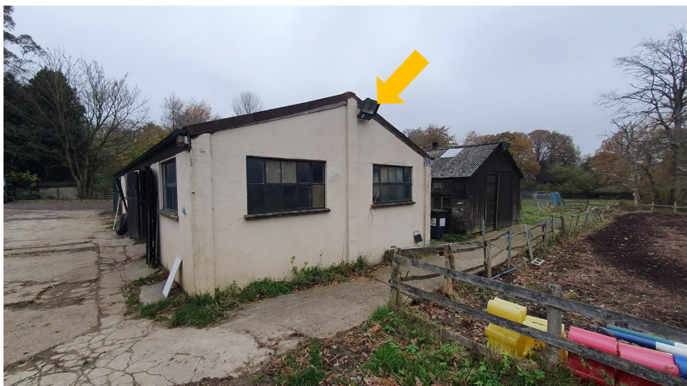
Photo 2. Existing stable - East elevation
